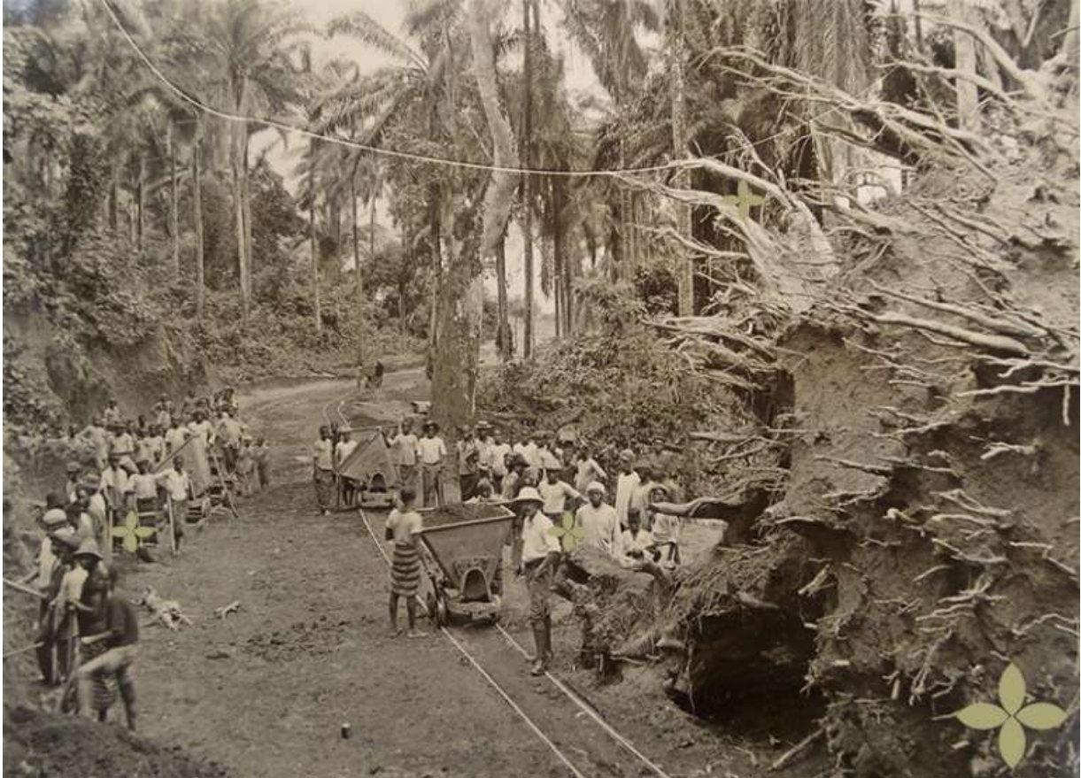
This photograph depicts the construction of Douglas Road in Owerri, Nigeria, in 1902. The project was accomplished through the manual labor of a large local workforce under colonial supervision. Photo credit; Ukpuru
