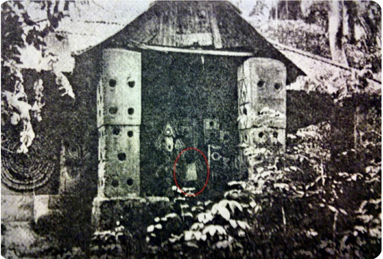
The largest single mbari structure still standing in 1966-67. – Herbert M. Cole, 1982.
