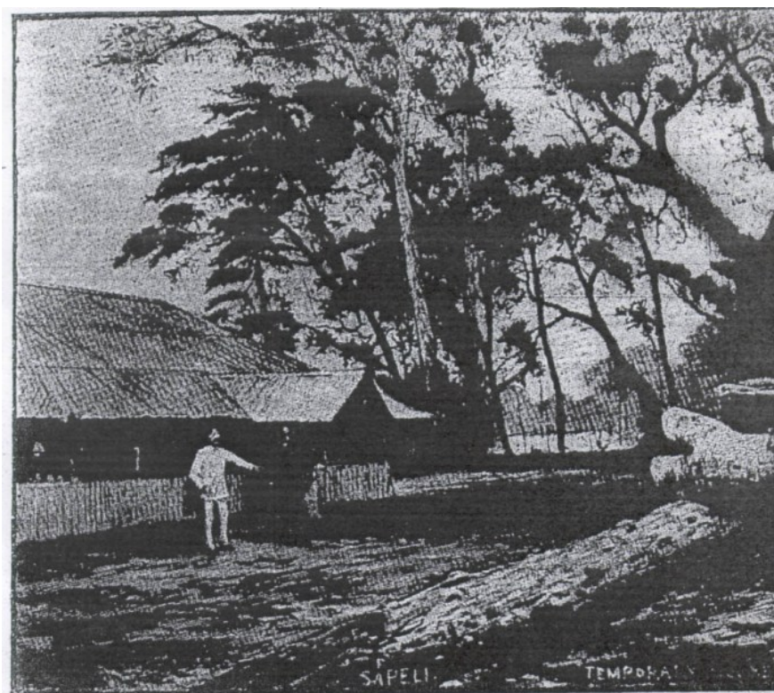
A Temporary House at Sapele
