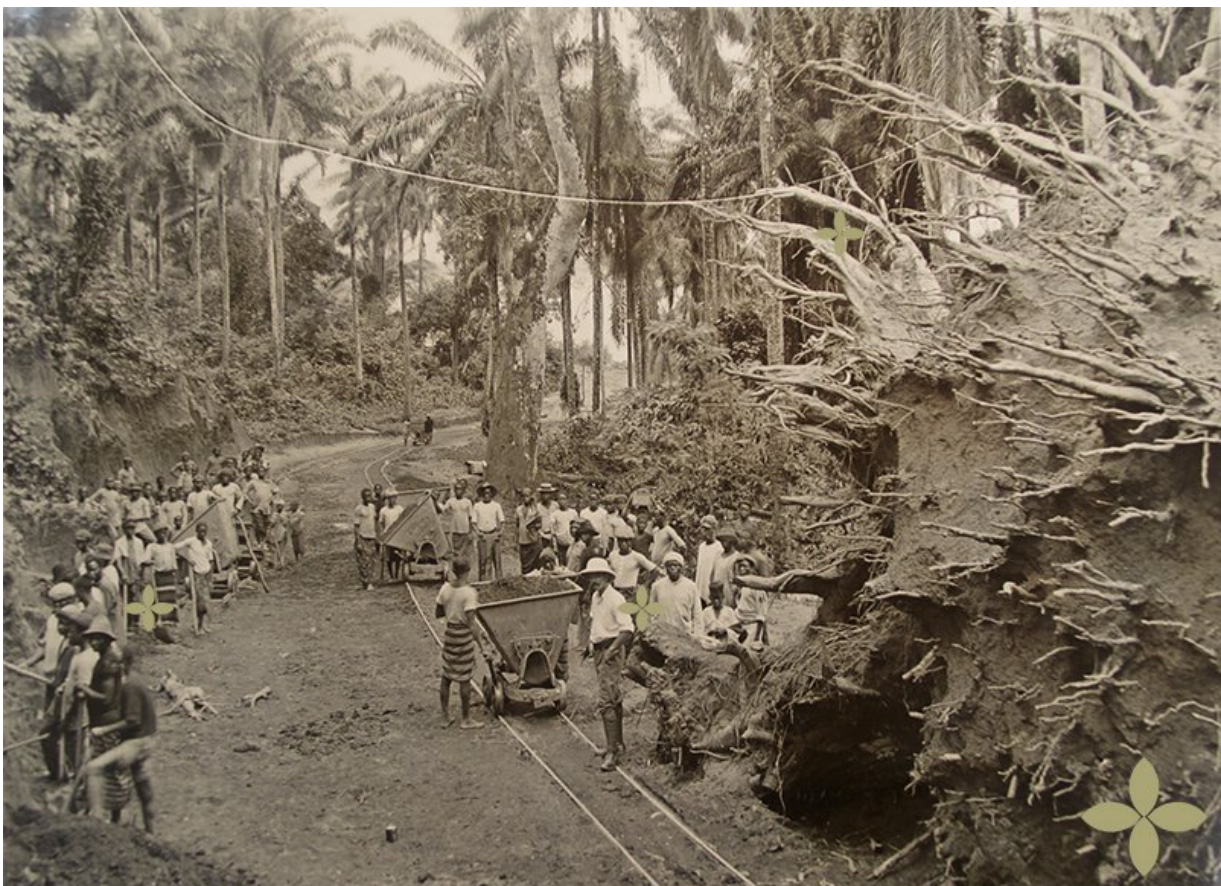
"Road making at Calabar." showcasing forced labour. c. 1909.
